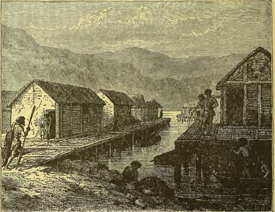
RESTORATION OF A LAKE SETTLEMENT NEAR THE SHORE.
